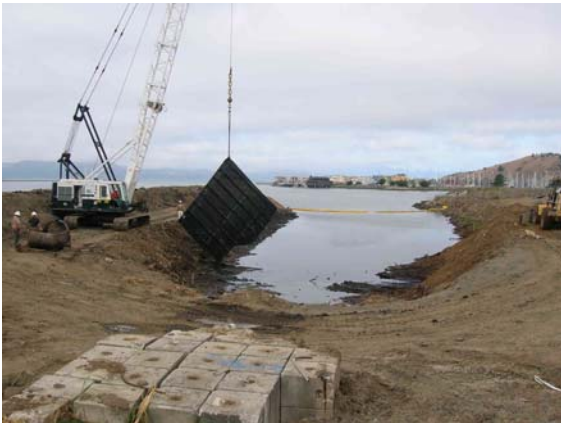
Figure 4. Removal of Ship Hull During Dredging Activities.
