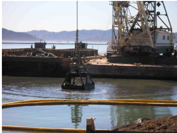
Figure 5. Positioning of Derrick Crane and Barge. Temporary Turbidity Barrier in Foreground
